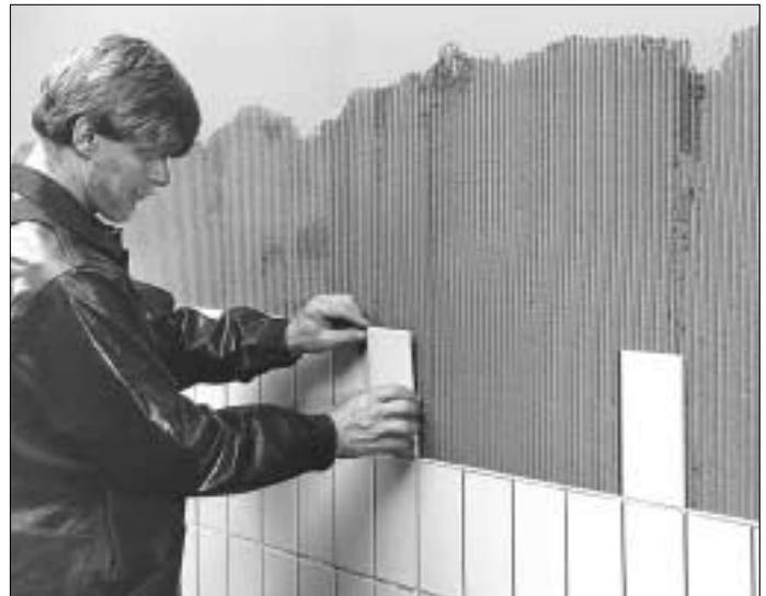
3. The tiles should be laid with spacing twine. Each tile should be pressed against the wall slightly to one side of the intended position and then twisted into place. To check adhesion, remove a few tiles immediately after fixing them. The backs should be completely covered with mortar. Take special care when bedding tiles with large profiles (studs or groves) on the back. Adhesive that has squeezed out more than half the joint depth is scraped off.
