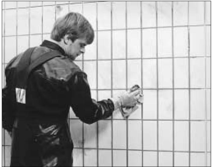
6. Final cleaning of clinker tiles with dry cotton waste within 15 minutes. Final cleaning for glazed wall tiles, use a stiff flat cellulose sponge, so that the grout in the joints does not come loose. After cleaning, keep the joints moist for about 3 days. On glazed tiles, the film of grout can normally be removed with a dry rag.
