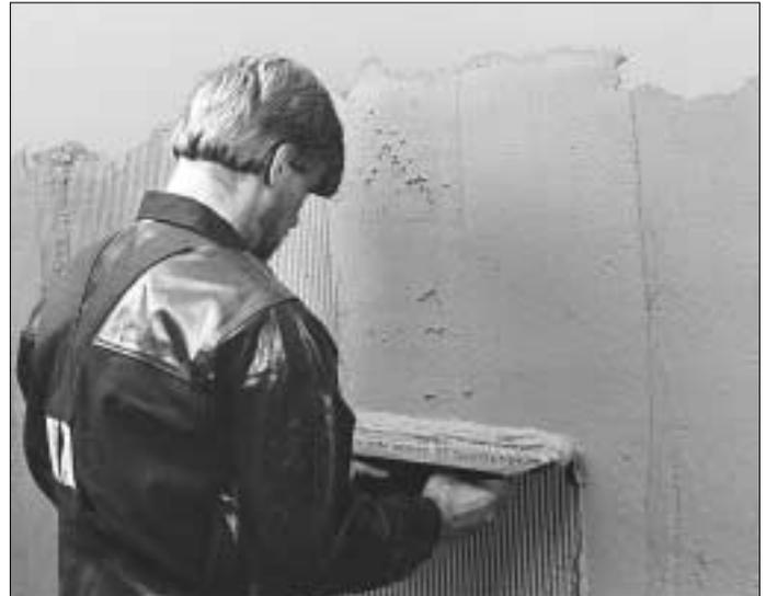
2. Then screed with a notched spreader held at right angles to the surface. **NOTE: Be sure to use the correct spreader according to the table.**
