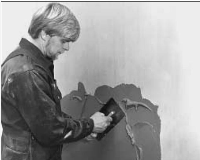
1. Spread the mortar with a trowel or spreader, working it well into the surface. Do not spread out more mortar than you can tile in approx. 10 minutes (FB14 - 5 minutes).
