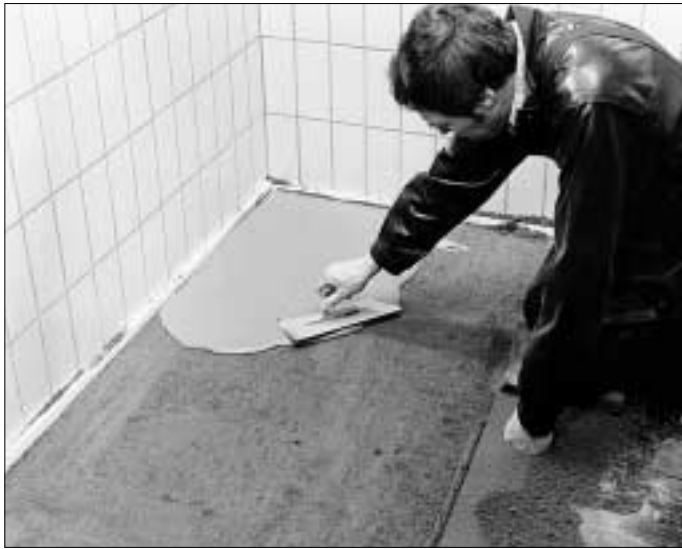
5. A fluid cement slurry (cement and water) should be spread over the bedding mortar.
