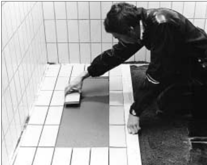
6. When the surplus water has been absorbed by the mortar and the slurry has taken on a matt appearance, the tiles should be laid out according to the markings on the gauge float.
