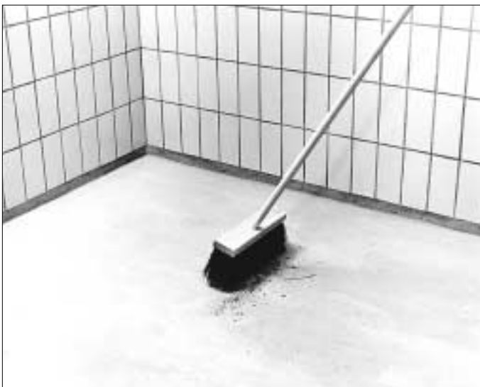
1. The sub-floor should be cleaned carefully before starting work.
