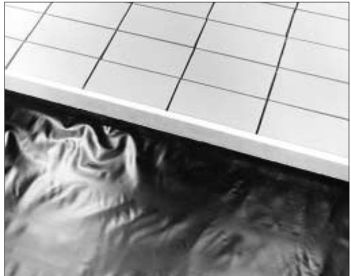
9. A strip of 10–15 mm cellular plastic should be laid along each expansion joint.
