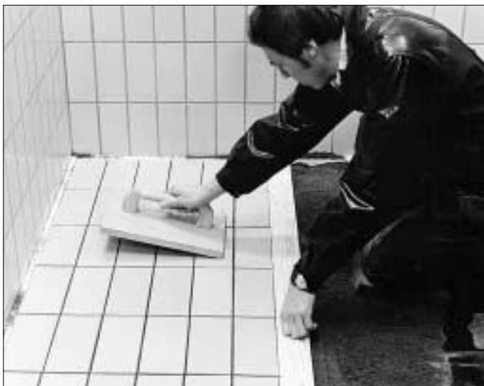
7. The tiles should be tamped down into the slurry.
