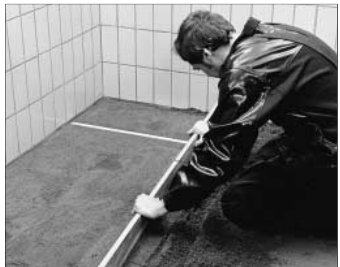
4. Position the guides at intervals of 2–3 metres, or at any other distance that is appropriate with respect to the area to be tiled. The mortar should be levelled at the right height according to the guides.
