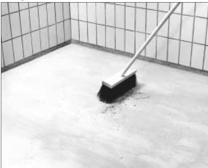
1. The surface should be cleaned thoroughly before starting work.
