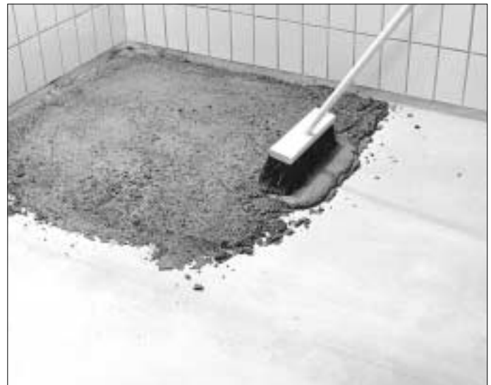
2. Cement slurry should be brushed into the surface immediately before the tiles are laid.
