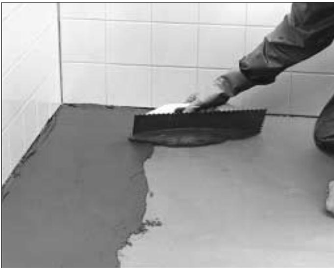
1. Spread the mortar with a trowel or spreader, working it well into the surface. Do not spread out more mortar than you can tile in approx. 10 minutes
