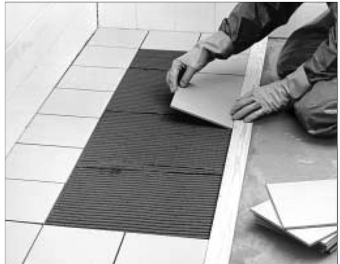
3. Position the tiles according to the marks on the gauge float and press the tiles firmly into place. The position of the tiles can be adjusted up to 15 minutes.
