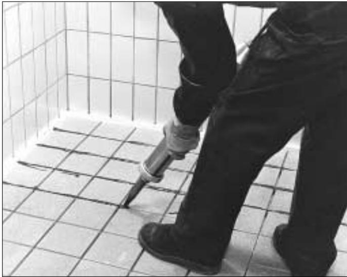
5. Apply the grout according to the respective product instructions i.e. with a gun, trowel or in accordance with slurry method. Remove as much grout as possible from the surface of the tiles.
