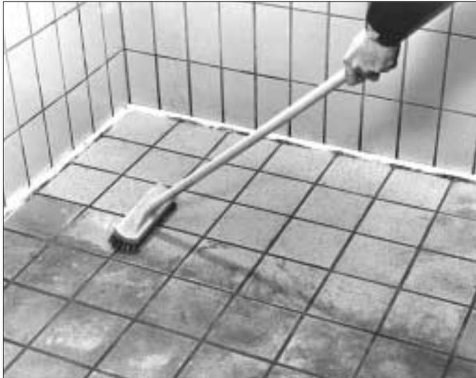
6. Allow a minimum of 24 hours after grouting before cleaning is commenced. Earlier cleaning will discolour the joints. Flush the floor with water sufficient to keep the floor damp for about 2 hours. Clean the tiles with a cleaning machine with rotating scotchbrite. Smaller areas can be cleaned with a scotchbrite (pad) or a hard brush. It may be necessary to remove spots of excess grout by using a steel spatula.
