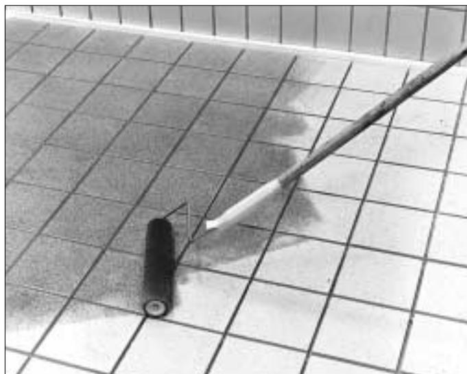
4. The tiles shall be treated two times with 2 hours drying time (at +20°C with good ventilation) between the treatments. The first treatment with uncoloured mixture and the second treatment with coloured mixture. Apply the mixture diagonally across the tiles. Move the roller gently without pressure to prevent the mixture flowing into the joints. Let it dry.
