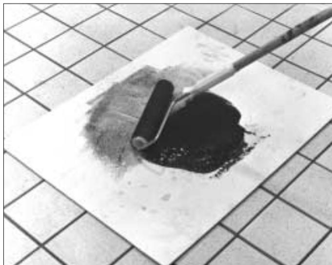
3. The application of the mixture shall be done with a short-haired roller – a so called mohair roller. Pour a suitable quantity of the mixture on a waxed paper. Rub a suitable quantity into the roller.
