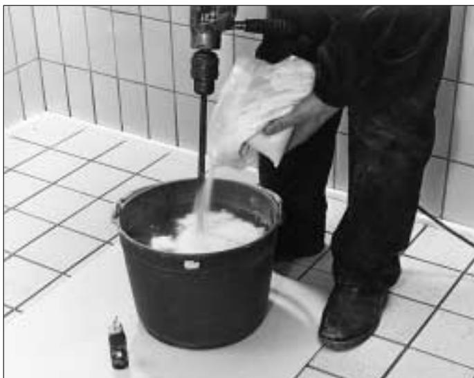
2. Mix the wallpaper paste in accordance to the directions given on the package. Normally 0.5 kg wallpaper paste to 5 l lukewarm water. Mix one uncoloured mixture and one coloured mixture (10 ml colour pigment to 5 l water). The mixture has to swell before the mixture is applied. We recommend the mixture to be prepared the day before it shall be used.
