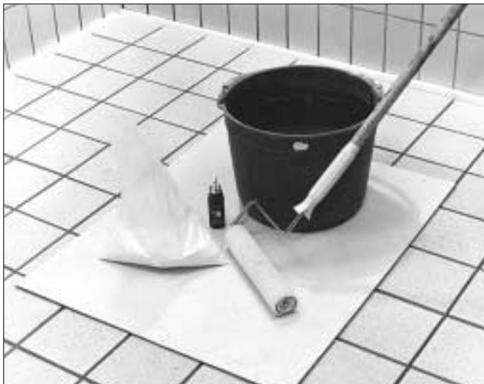
1. The coating consists of water soluble wallpaper paste, water and water soluble colour pigment.
