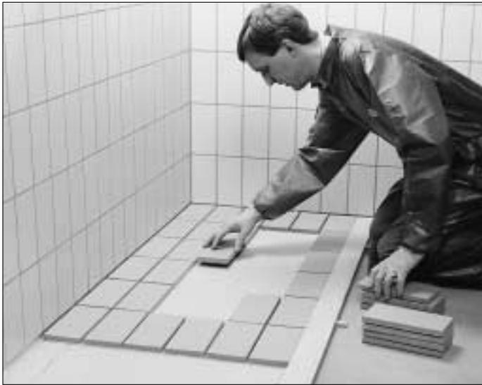
5. Lay out the tiles according to the markings on the gauge float. Press the tiles lightly into the adhesive compound. Use spacer blocks on the underside of the gauge float to keep it out of contact with the mortar.
