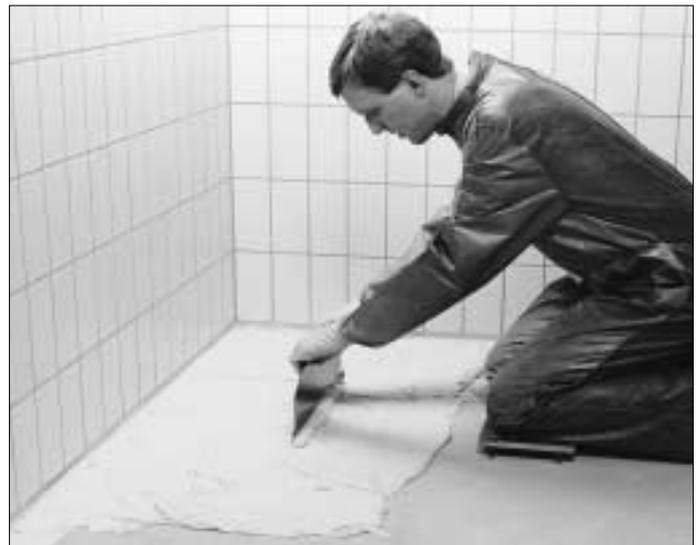
4. Even out the layer of compound with a trowel that generates a thickness of 4 mm. The compound should swell somewhat against walls and previously laid tile courses. The surface of the layer of compound should be free of holes and depressions.
