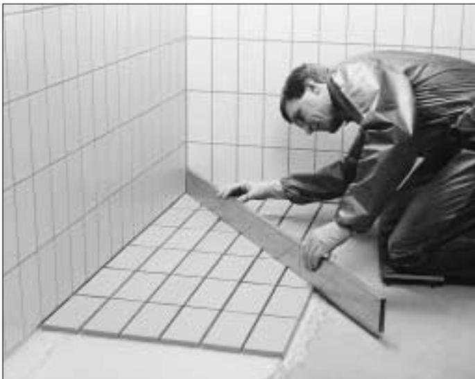
6. The evenness of each newly laid surface should be carefully checked with a gauge float. If adjustment is necessary, a tile can be lifted with the aid of a bent nail. Tiles should be adjusted within 5 minutes after they have been laid. If the laying process is interrupted, excess adhesive compound along the edge of the tiles should be removed with a spatula or similar tool. The floor should be closed to traffic for about 24 hours, after which joints can be filled.
