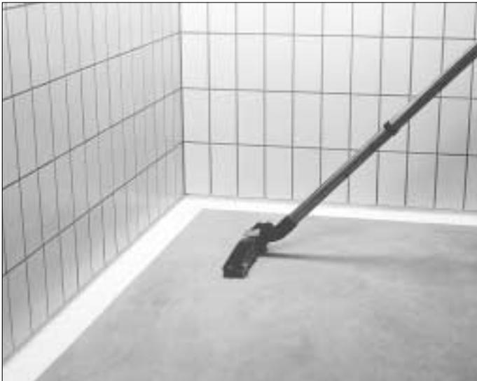
1. The surface must be free from paint, grease, loose particles and dust. Sweep and vacuum clean the floor thoroughly before starting work.
