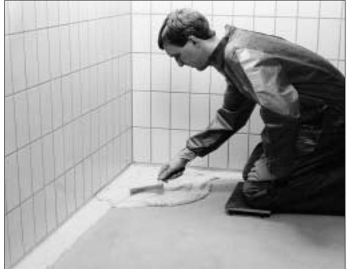
3. Spread the compound on the surface with a steel float or similar tool. The layer of compound should be 4–6 mm thick.
